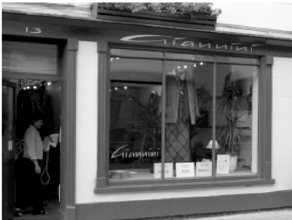
A fine example of a traditional shopfront
